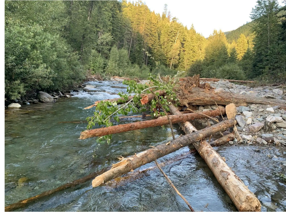
Placed wood structures and rock create instream complexity in the Vermillion River, Montana
